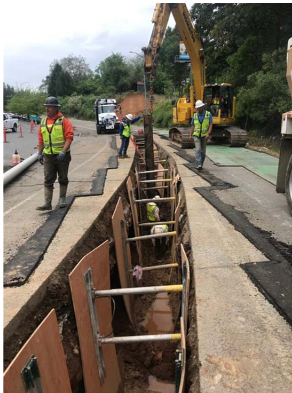
Sewer main replacement work as part of the Upper Broadway Bike Lanes Project, funded by Measure H&L!
